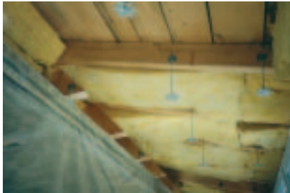
The roof construction was insulated inside with 200 mm ISOVER glass wool between the rafters and the mounting system Rosatwist.
