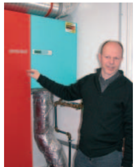
Comfort Ventilation Systems with integrated heating and hot water supply are available today as compact units that hardly need more space than a fridge. (Ing. Lang Consulting)
