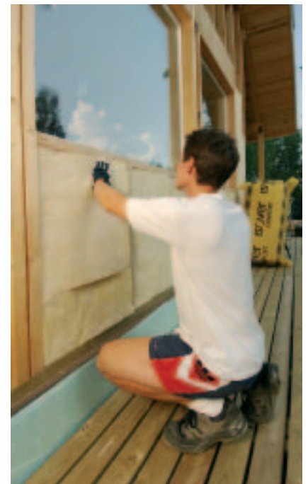
Filling the wood-frame construction tightly with ISOVER glass wool
